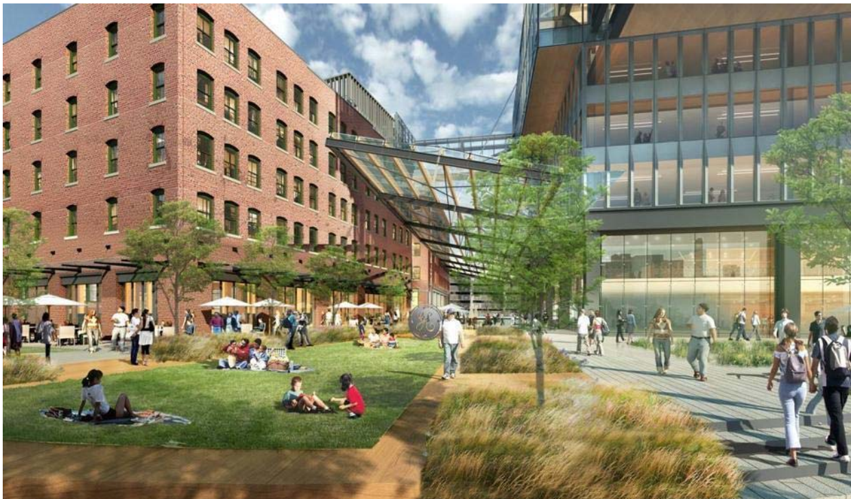
General Electric plans to renovate two brick building as part of its new headquarters in Boston's Fort Point area. A new 12-story tower is now slated to open in 2021.
