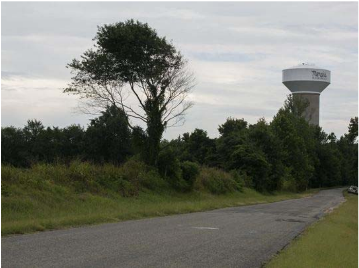
August 17, 2016 - The water tower in Stanton recently had "Memphis Regional Megasite" painted on top of the structure. Many West Tennessee businesses and leaders have pinned their economic futures on the Memphis Regional Megasite, which could produce 34,244 jobs.
