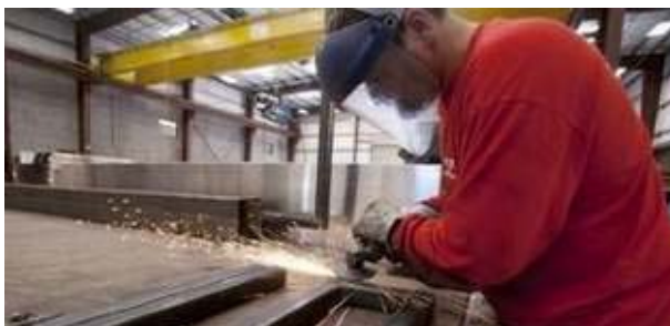
Purchase this Photo Young Electric Sign Company employee John Kovacs grinds a beam as he works to build a sign at YESCO's manufacturing facility at the Fort Pierce Industrial Park Wednesday in St. George. (Jud Burkett / The Spectrum)
